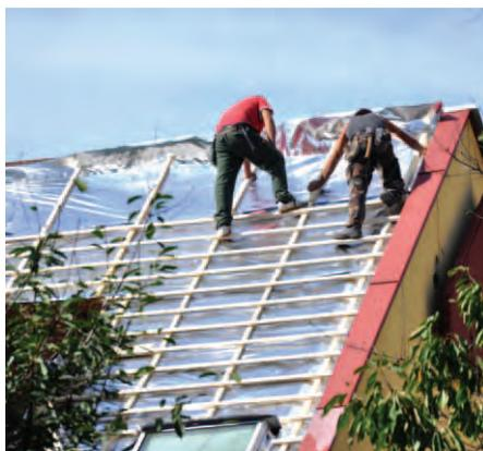
Various kinds of alufoil material are now on the market. One example is bubble foil insulation which uses a combination of reflective alufoil along with a single layer of bubble insulation or a double layer of bubble insulation to reflect heat.
